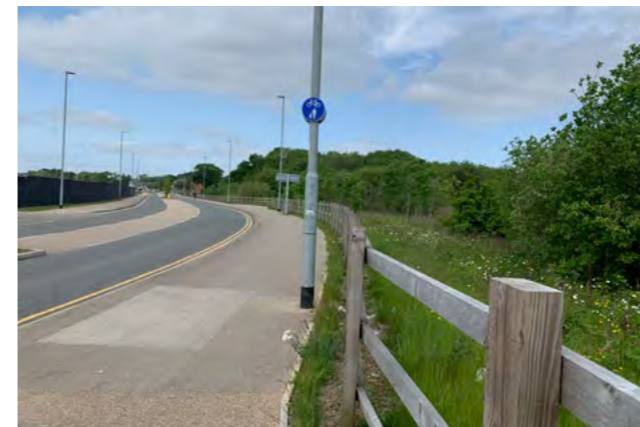
2 Existing timber fence boundary along Enterprise Way
