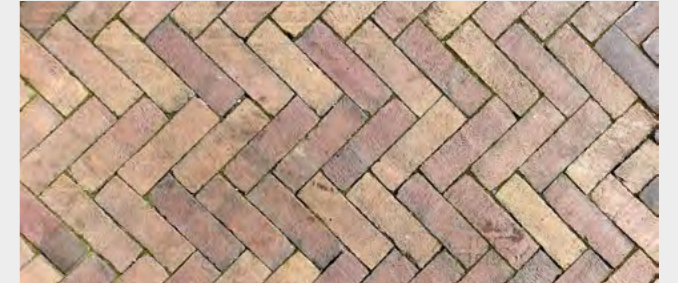
Clay paving - laid flexibly utilising SuDS build-ups
