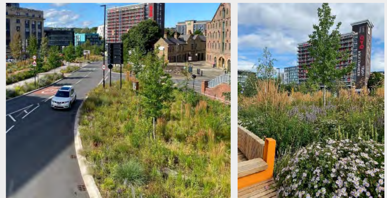
Indicative Photo of Bioretention Systems
