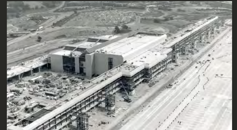
Manchester Airport Terminal 2 Development, 1993 Manchester Airports Group
