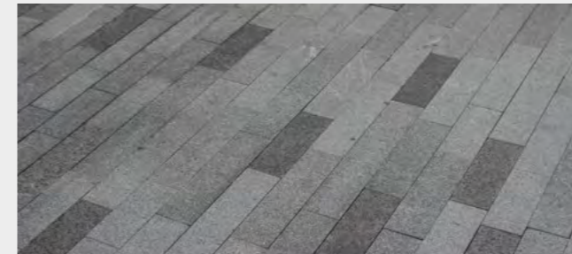
Concrete paving - Laid flexibly utilising SuDS build-ups
