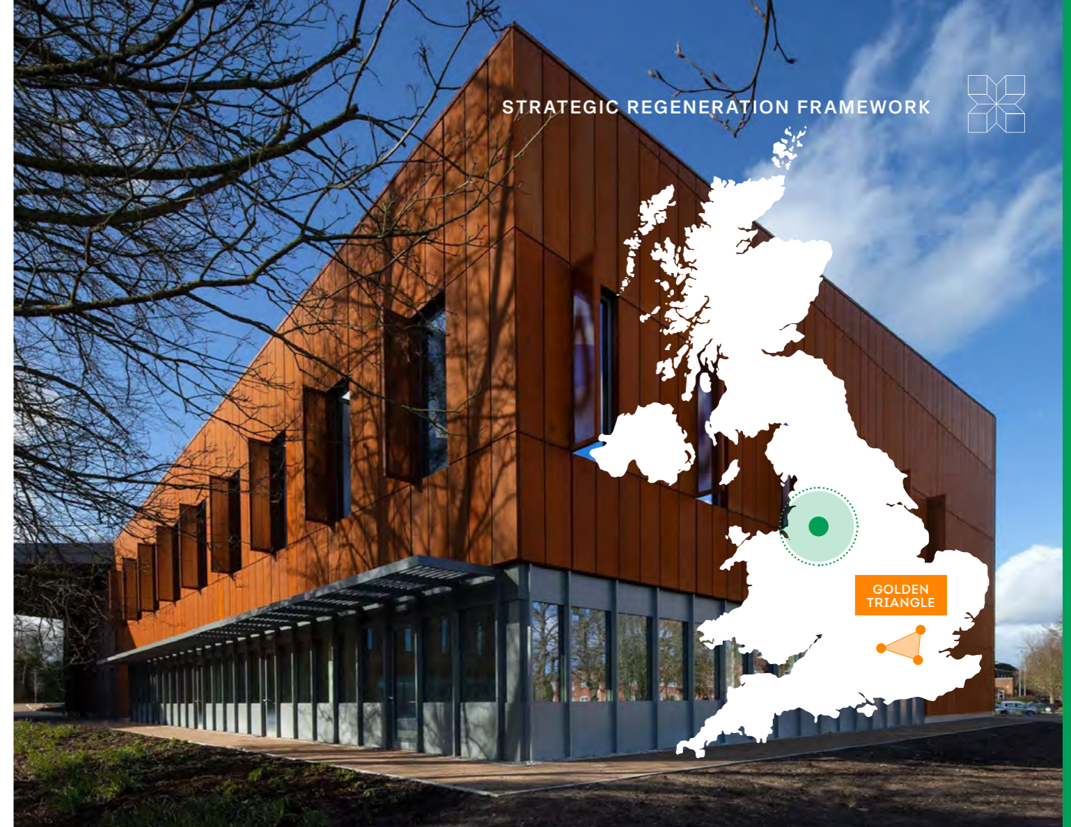
Zeus Building, Harwell Mid-Tech facility near Oxford Allies and Morrison Architects
