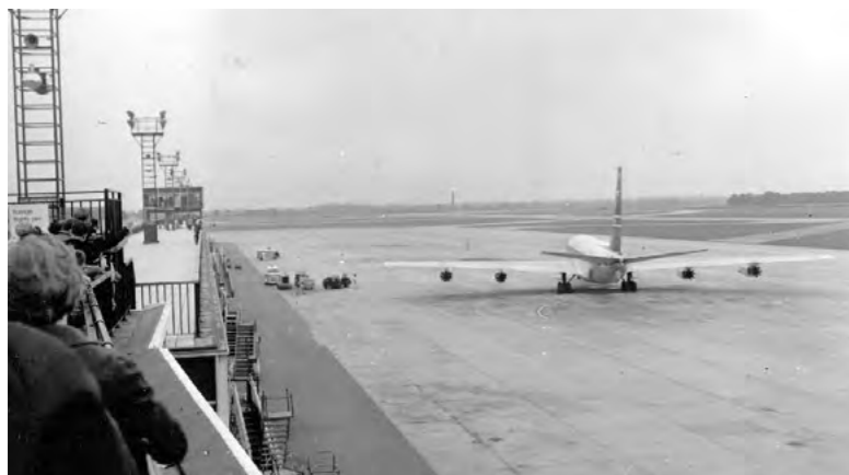
Ringway, Manchester Airport, 1962 Manchester City Council Local Image Collection
