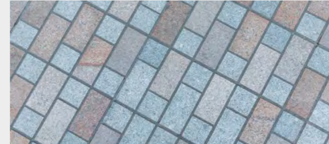
Natural stone paving - potential to explore permeable installation methodologies to not vehicular areas
